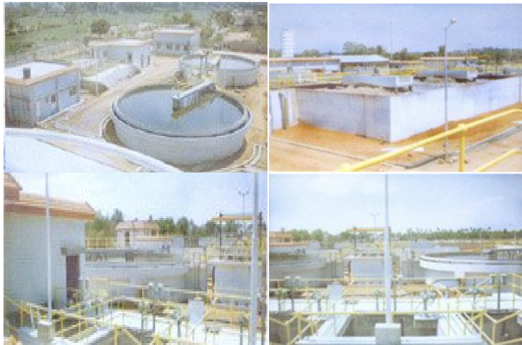
Figure 9: Photographs of 10 MLD Tertiary Treatment Plant (TTP) at Yelahanka, Bangalore
